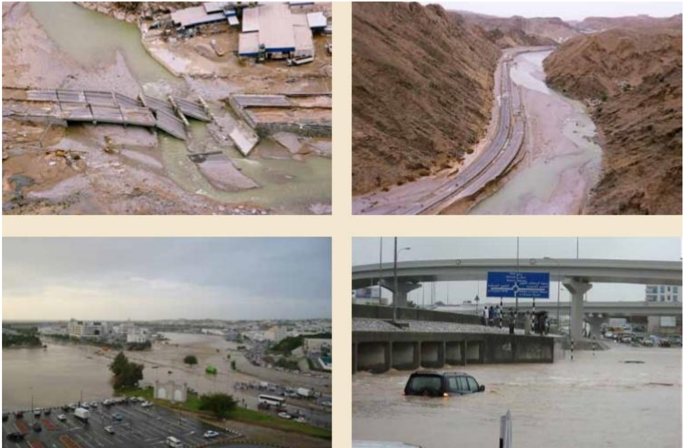
Figure 1. damage cause by floods
